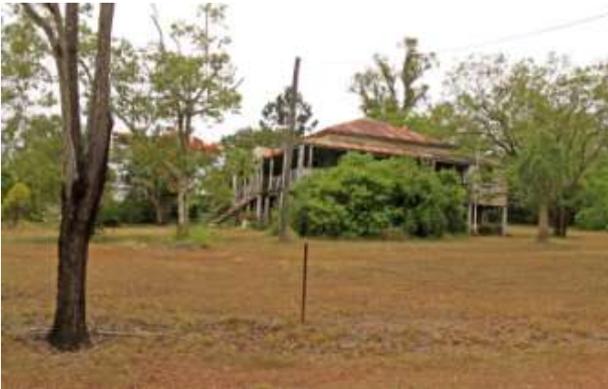
Abandoned farmhouse near Esk
