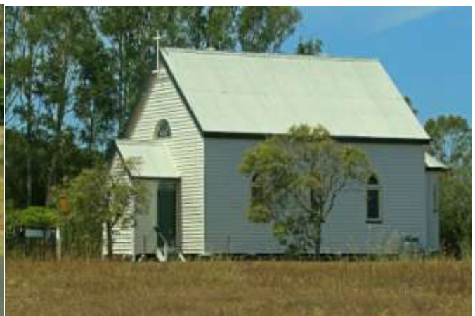
This old church is now someone's home
